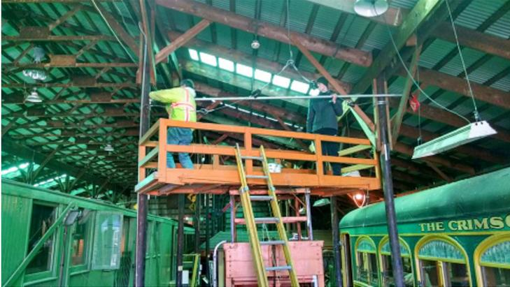
*Charlie Lowe and Todd Consadine are on the tower car over Track 23 installing the compression pipe between the poles.*
