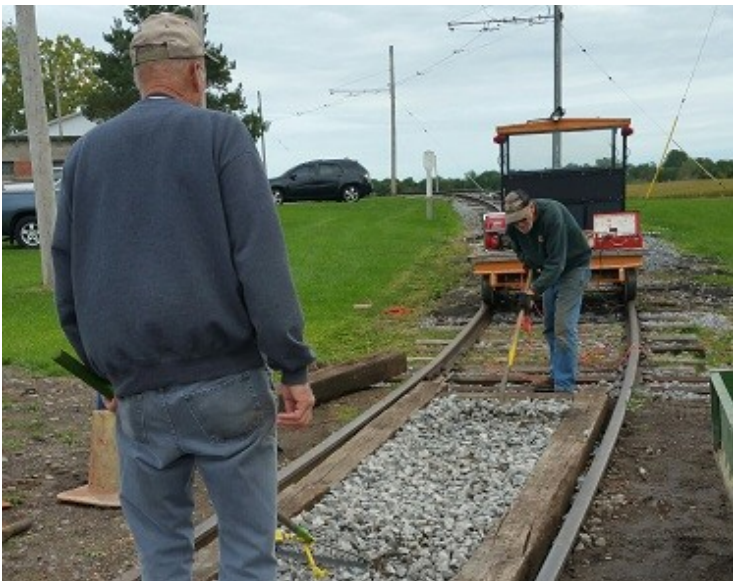
Rick Holahan is ready with the rake as Taylor Reed shovels more ballast in the Forest Lane Crossing. Photo by Rich Fischpera
