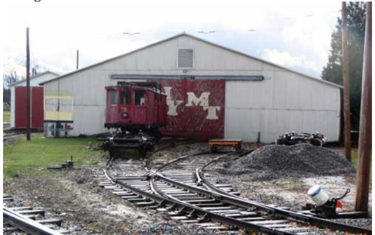
The switch is complete and track 23 is ready to march into the barn, as line car 2 looks on. Charles Lowe photo
