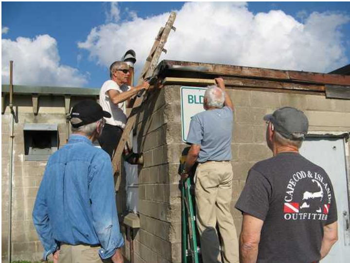
Don Quant and Bob Pearce deal with rotted wood and rusted flashing as John Ross and Jim Moe offer moral support.
